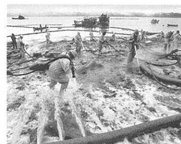
High pressure and hot water treatment being used to clean up the Exxon Valdez oil spill
