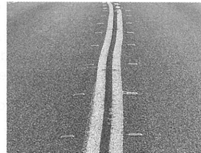
Cat's eyes are reflective road markers that glow at night to guide motorists.
