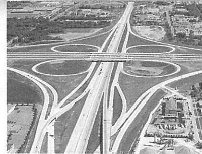
A cloverleaf interchange helps in the non-stop flow of traffic where two highways cross.
