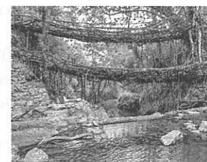
In Meghalaya, the prop roots of rubber trees are guided to grow across wooden frames to form living bridges.
